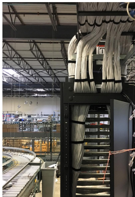
Cable tray and ladder mount installed at Personal Creations, Inc.
