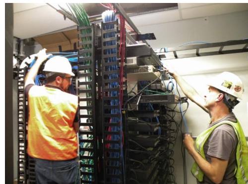
NexGen techs cross-connecting cables to the data network infrastructure
